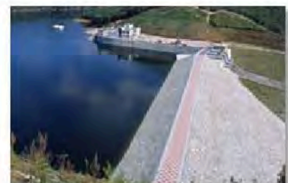
Dam construction / monitoring
